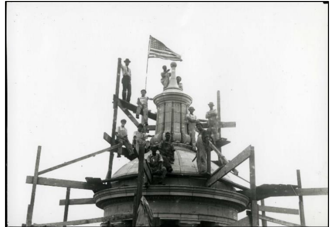
Image: Building the cupola on Plainfield City Hall. Photo by Paul R. Collier, 1917.
